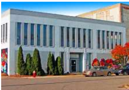
THE PONY RIDE BUILDING 1401 VERMONT AT PORTER IN THE CORKTOWN NEIGHBORHOOD OF DETROIT
